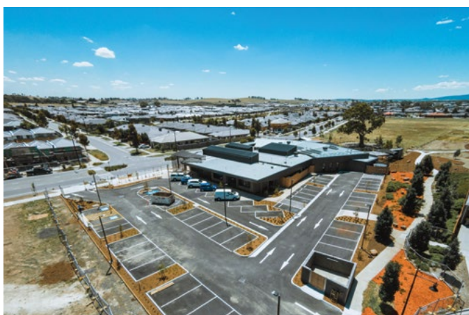
External lighting, Jindi Family and Community Centre (City of Whittlesea)
