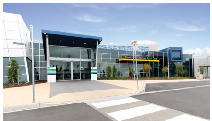
Entrance accessible to all modes of transport, Thomastown Recreation and Aquatic Centre (City of Whittlesea)
