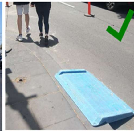
FIGURE 23: PROVIDE TEMPORARY RAMPS FOR MOBILITY IMPAIRED AND WHEELCHAIR USERS
