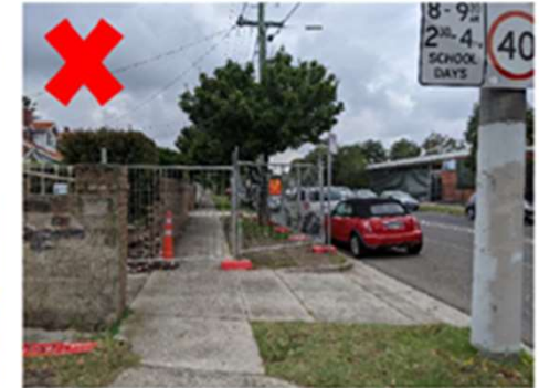
FIGURE 9: NO CLEAR ROUTE EXCEPT IN ROAD - ENSURE CLEAR, LEGIBLE ROUTES FOR PEDESTRIANS IF THE FOOTPATH IS CLOSED
